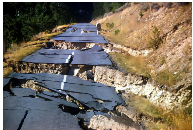
Hebgen Lake Earthquake Damage
